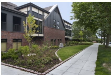
Exterior View from Street
