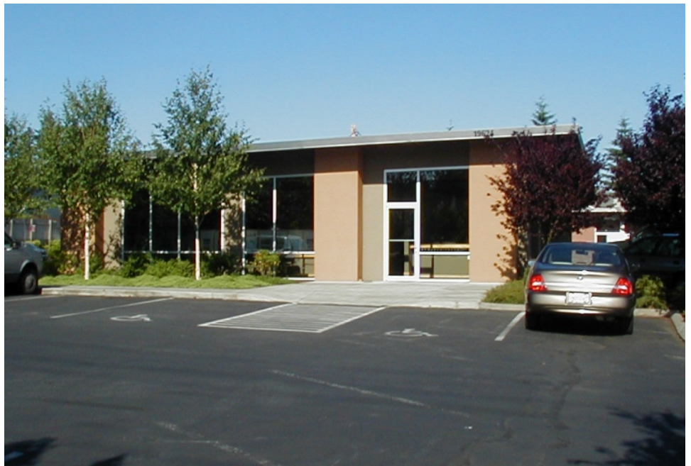
Exterior View Of Renovation
